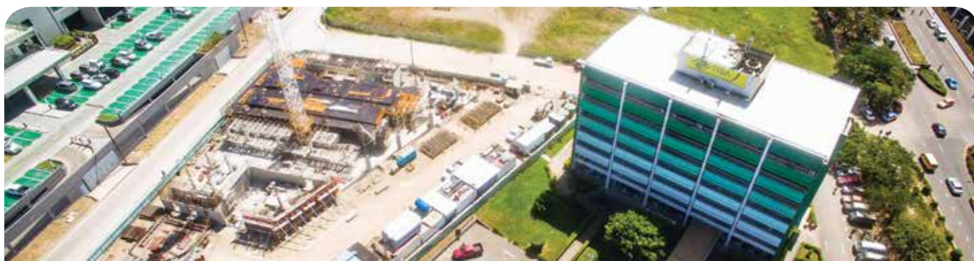
Aerial view of the TISA Rua construction.
